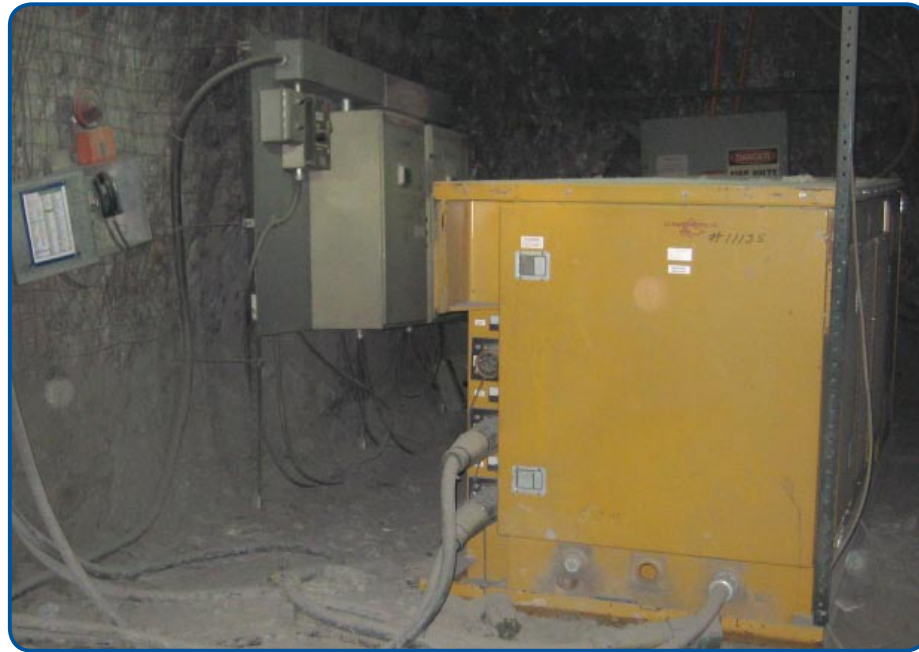
Figure 1: Telephone Station in Underground Mine
