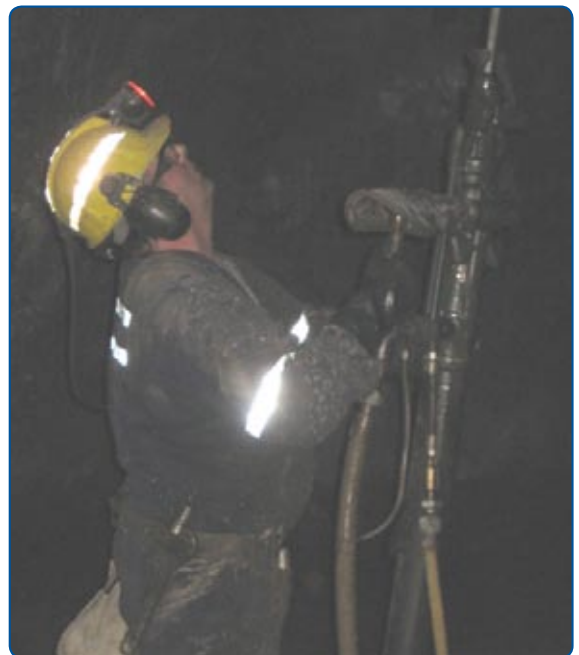
Figure 4: Operating a Stoper to Drill Hole Overhead
