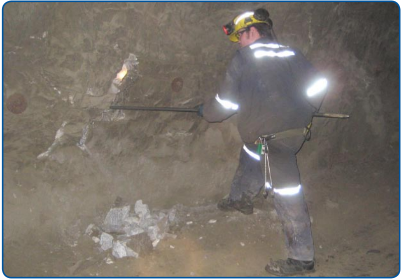
Figure 1: Scaling Wall of a Drift
