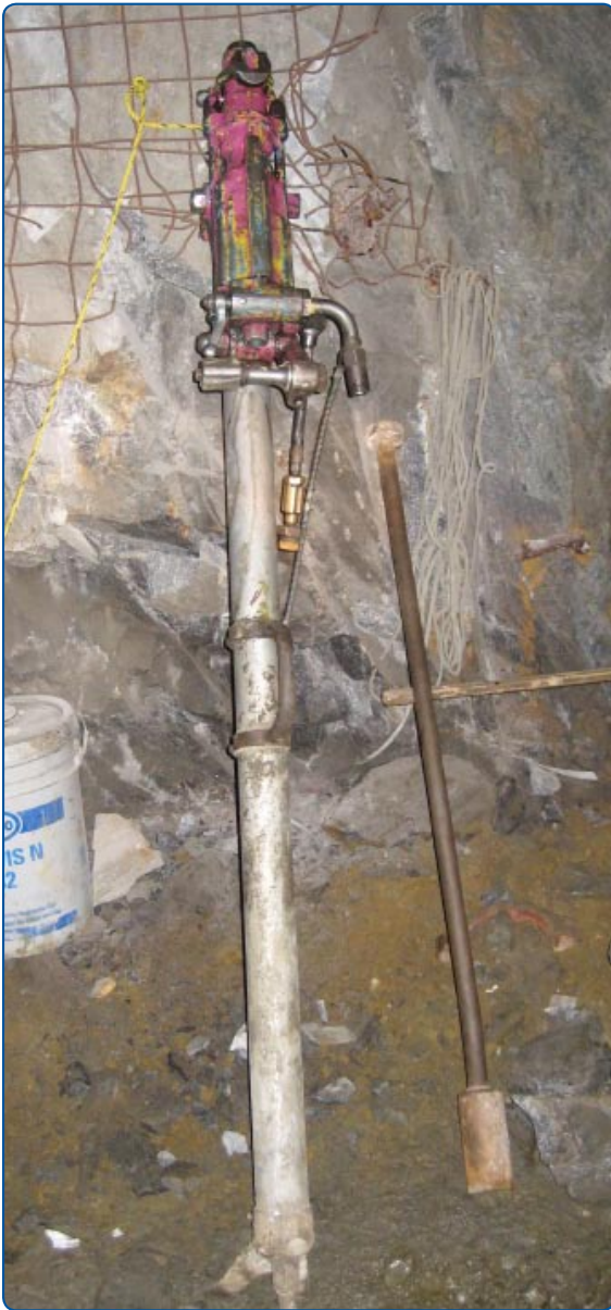
Figure 1: Jackleg Used in Order to Install Platform for Slusher
