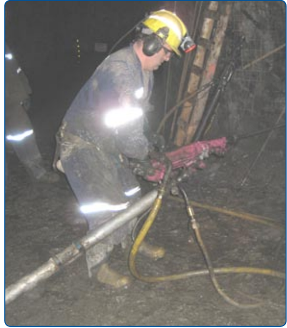
Figure 2: Operating Jackleg to Install Bolts
