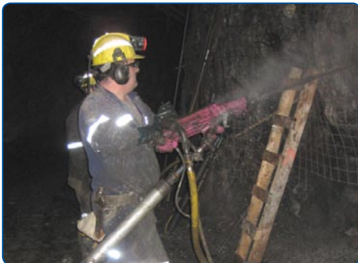
Figure 3: Operating a Jackleg
